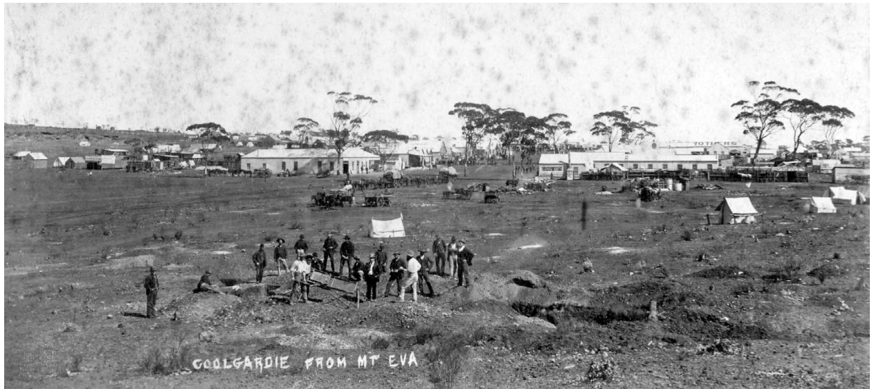
Figure 4. Photograph taken probably in 1894 looking west-southwest across Fly Flat towards Coolgardie. Note shallow excavations in foreground and dry blowing or shaking table within the group of men. The road to the newly discovered Kalgoorlie goldfield passes out between the buildings and to the left (with two horse-drawn wagons setting out). The caption is incorrect: Mt Eva lies some 500 m north (to the right) of the vantage point. Used with permission of the Coolgardie Goldfields Exhibition Museum.
