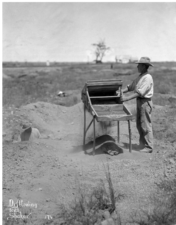
Figure 6. Miner dry blowing with screen and shaker. Location unstated, but within the Eastern Goldfields and possibly near Coolgardie. Sieved dry soil or sand is placed into the back, then a rocking motion causes it to pass forward and downward on a sloping platform with lodgement of the heaviest particles behind the cross-wise riffles. The operator would pause periodically to empty out the gold-bearing material from behind the riffles. Any large nuggets are picked off the screen. Sophisticated models also incorporated foot-operated bellows to blow out the light particles and fluidise the soil. Used with permission from the State Library of Western Australia (Call No: 010178PD).
